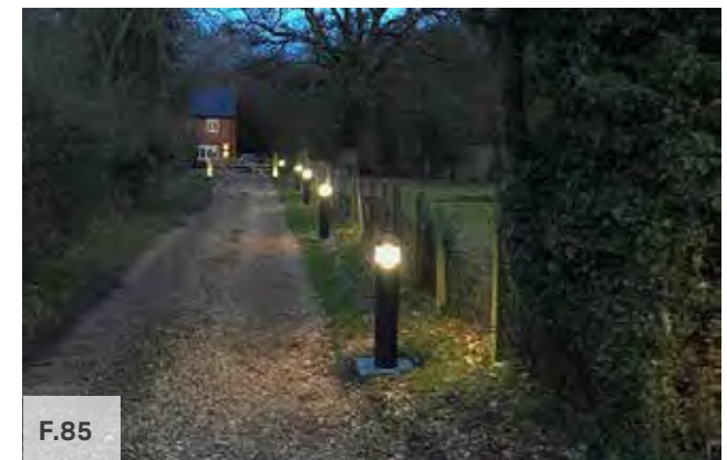
Figure 85: A negative example of lighting pollution on Common Lane as it is illuminated from early dusk to late dawn. A PIR movement sensor and a light fitting that prevents the light spilling vertically would be more appropriate. (Source: Binfield Heath Parish Council)
