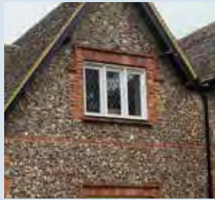
Multi leaded casement window with red brick inlet as decoration
