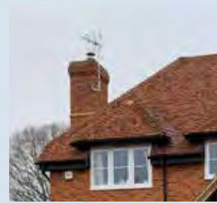
Plain tile and red brick chimney stack
