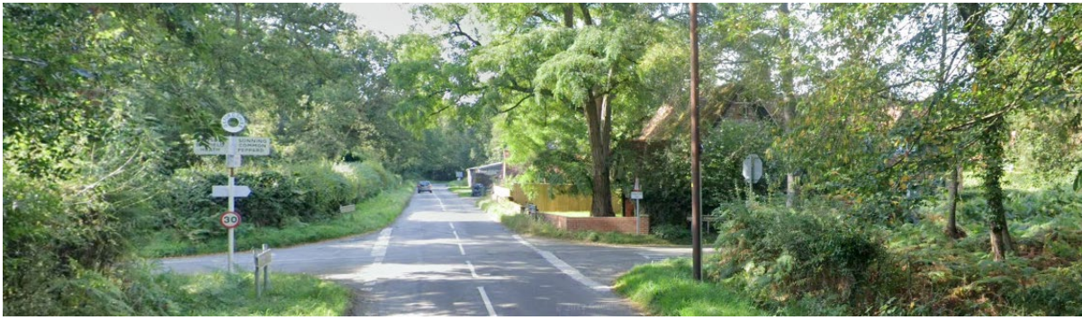
Figure 24 Coppid Crossroads, where Emmer Green Road meets Harpsden Road. Much of the road network is heavily lined with trees
