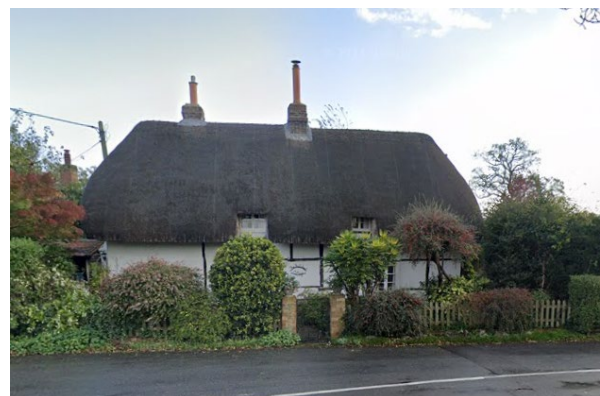
Figure 5 The Thatched Cottage - 17th Century, Grade II Listed Building
